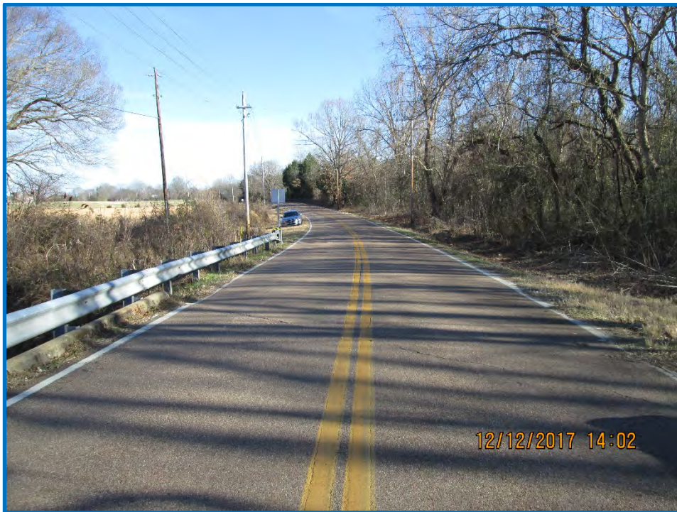
Looking east standing near middle of bridge
