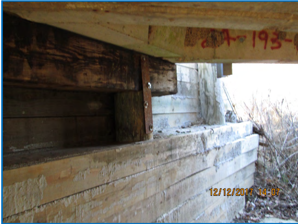
Looking at west abutment standing under bridge
