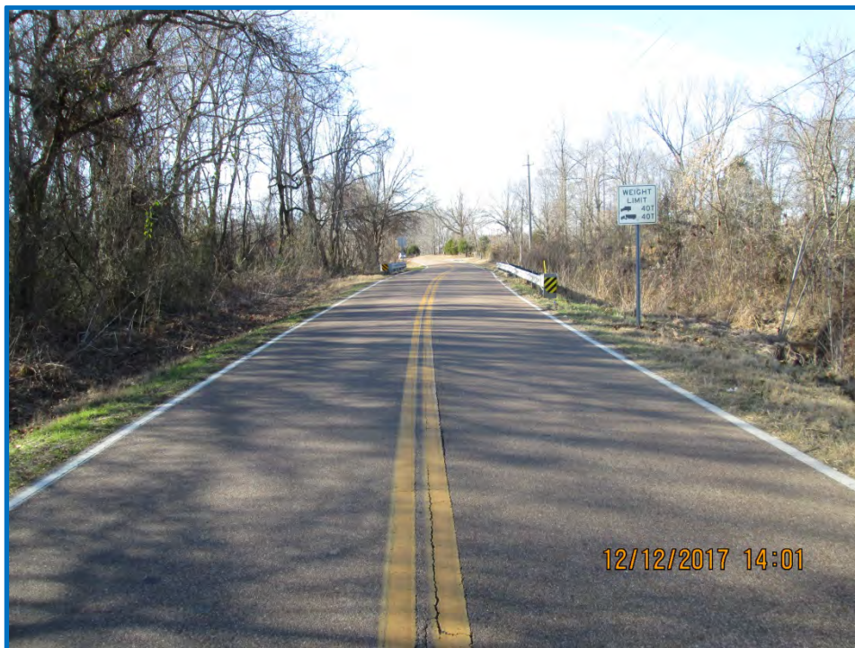
Looking west across bridge
