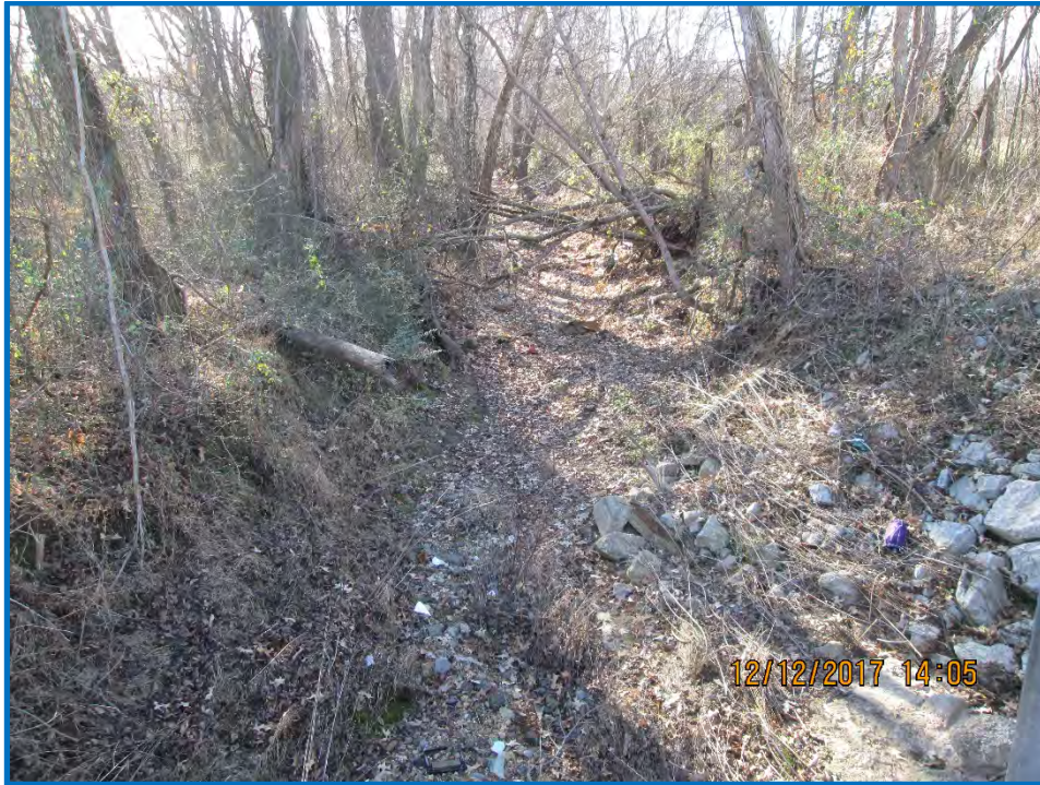
Looking south at downstream side standing on bridge
