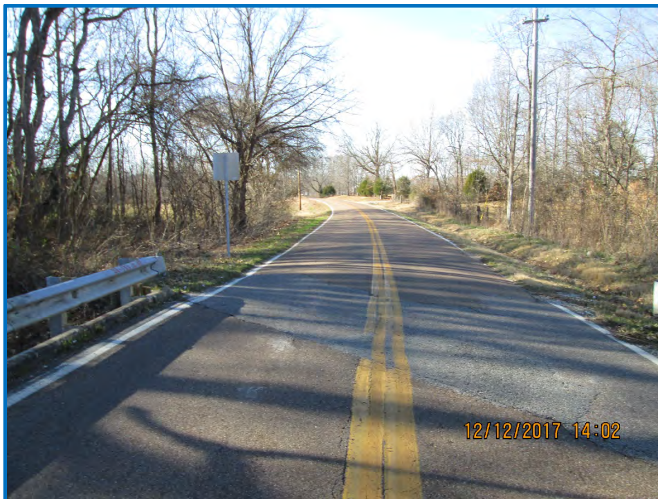
Looking west standing near middle of bridge
