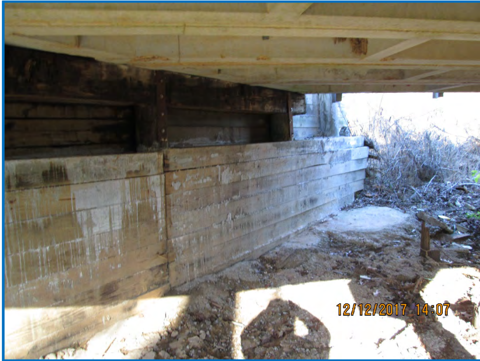
Looking at west abutment standing under bridge
