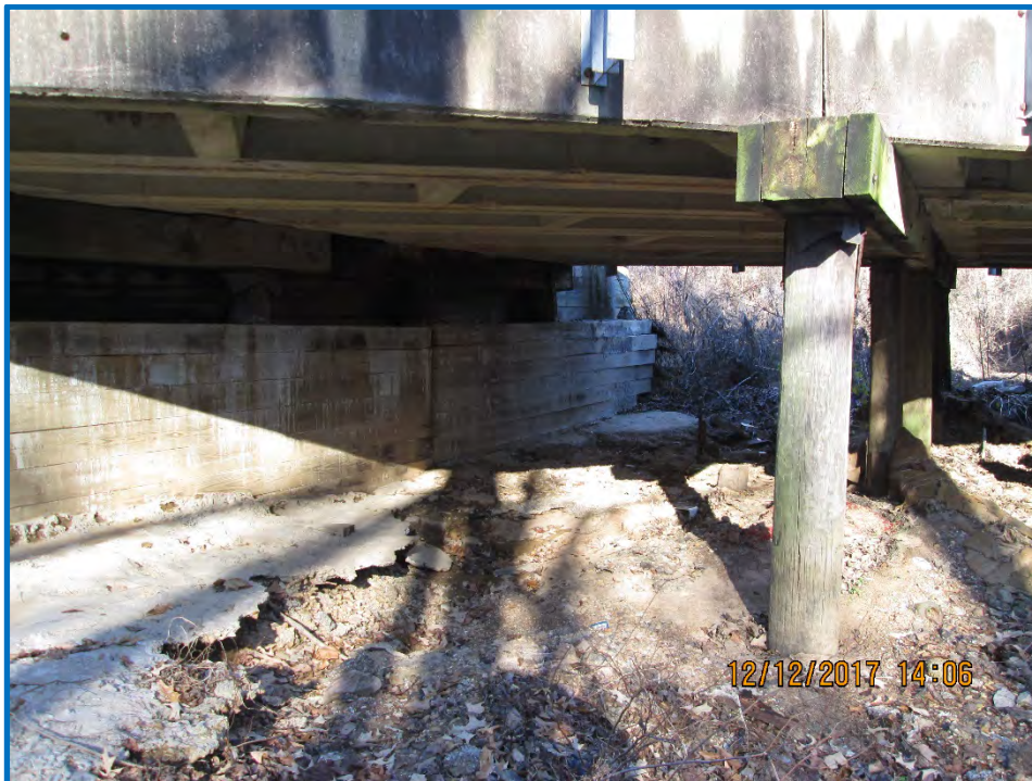
Looking at west abutment standing on the south side of bridge
