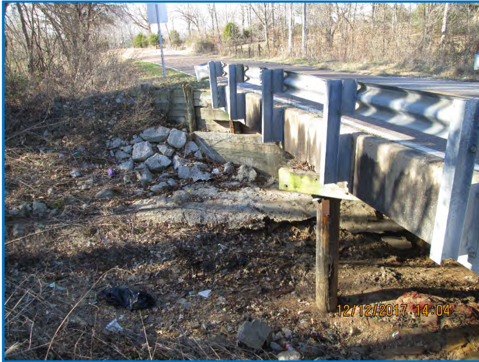
Looking at downstream side standing off SE corner of bridge
