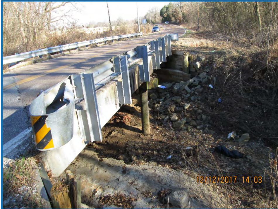
Looking at downstream side standing off SW corner of bridge
