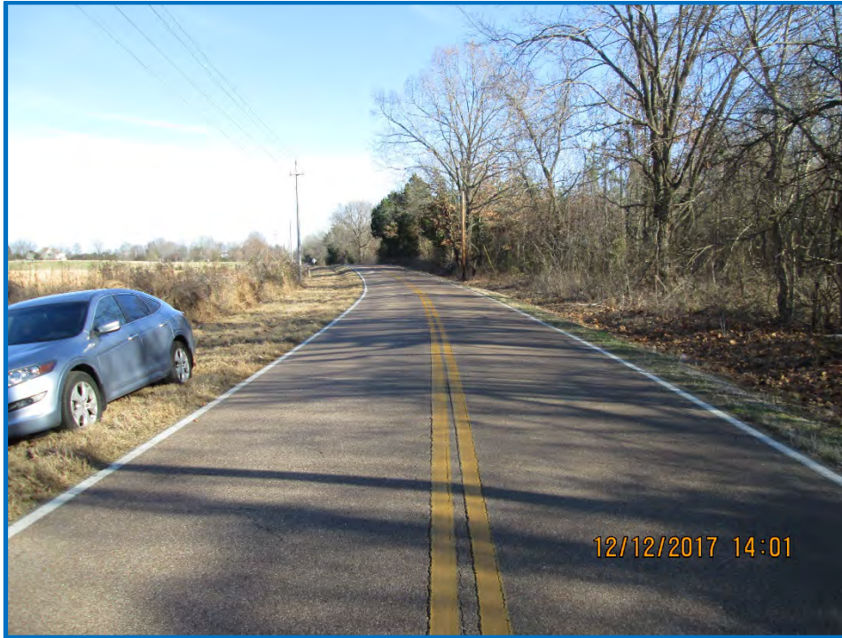
Looking east standing off east end of bridge
