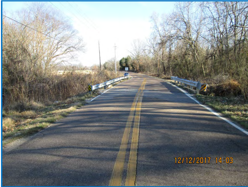
Looking east across bridge standing near west end of bridge
