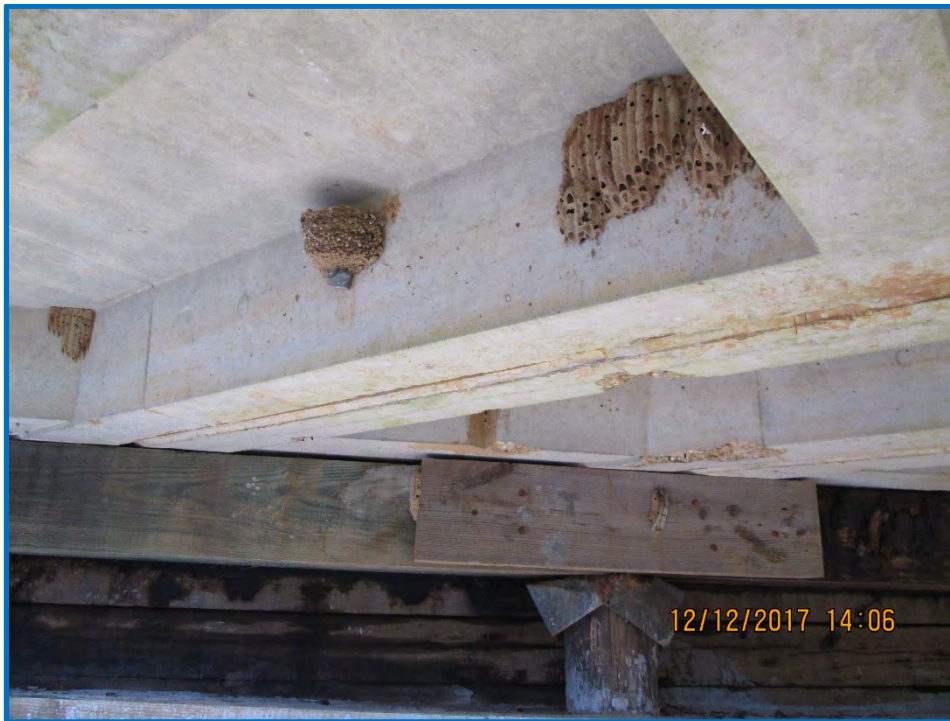
Looking under bridge deck
