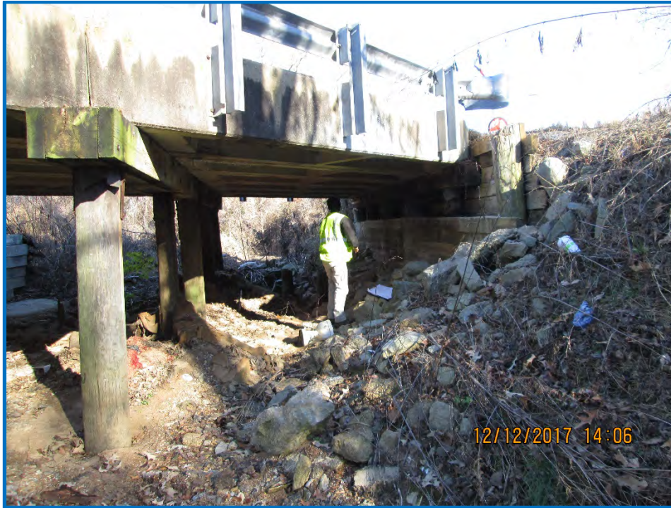
Looking at east abutment standing on the south side of bridge
